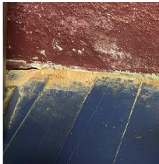
Interior stucco damage at interior
