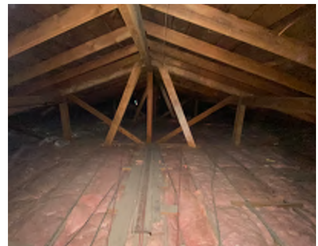
Overstressed framing and 6" insulation in attic
