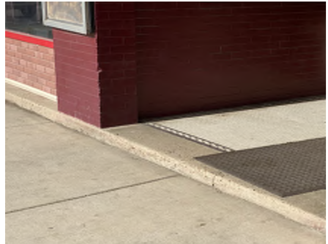
Front entries not accessible (tripping hazard)
