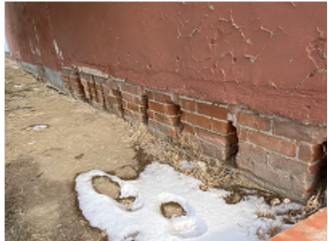
Negative drainage, voids, and masonry damage
