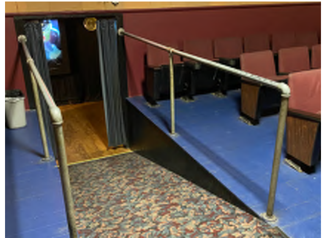
Non-compliant ramp and guards at Theater
