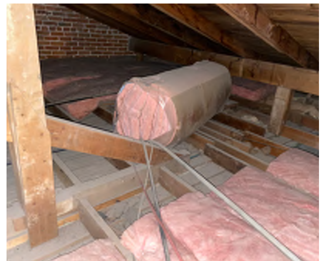
Insulation/venting/framing issues in attic
