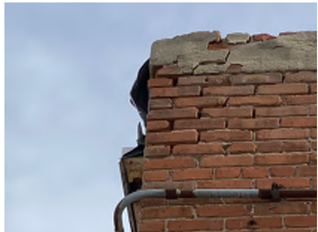
Parapet deterioration and waterproofing issues
