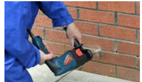
Drilling holes for damp-proof course injections
