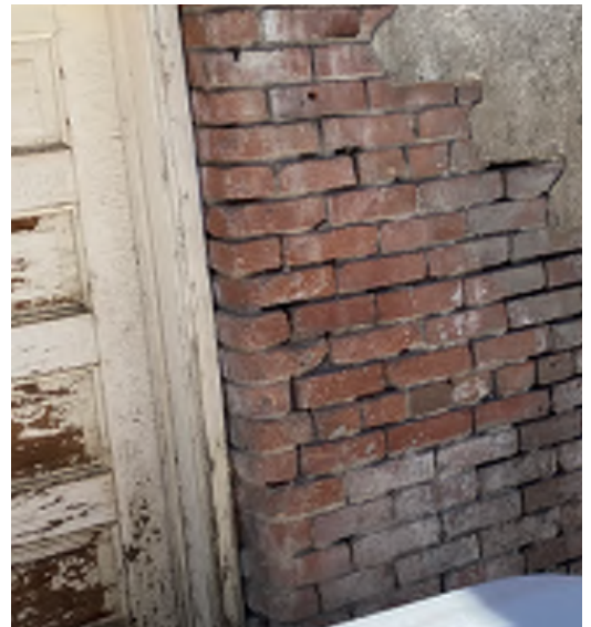
Rising damp damage at brick/stucco
