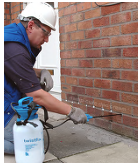
Injecting curing damp-proof product
